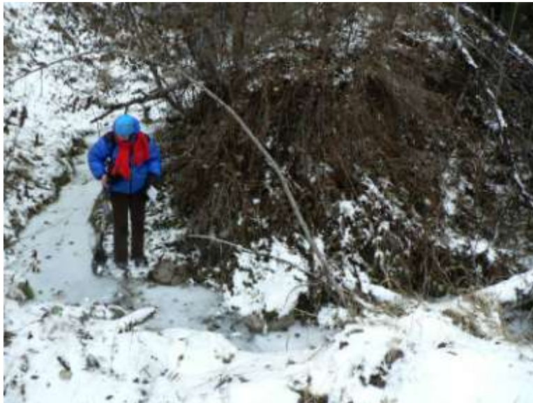
Figure 4: Breach of Swift's Ditch—ie. the Blow Out (2009)
