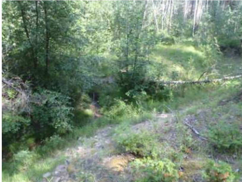
Figure 5: Breach of Swift's Ditch—the Blow Out (2010)
